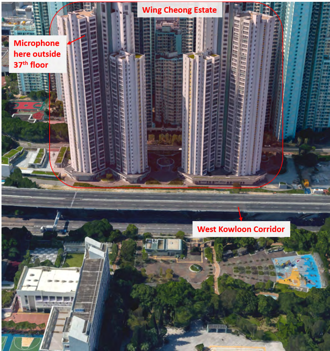
Figure 5.1: Google Earth's 3D-viewer snapshot, showing the measurement's physical environment and the microphone's 37th-floor location.
