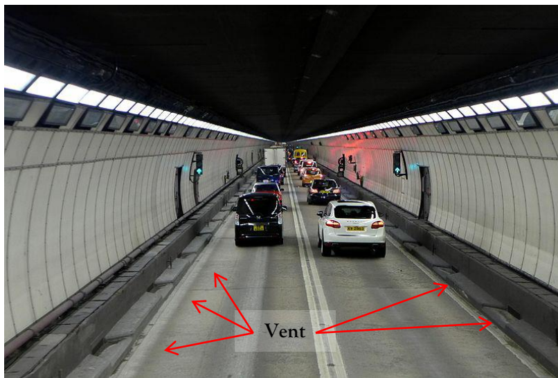
(b) Photo of the tunnel
