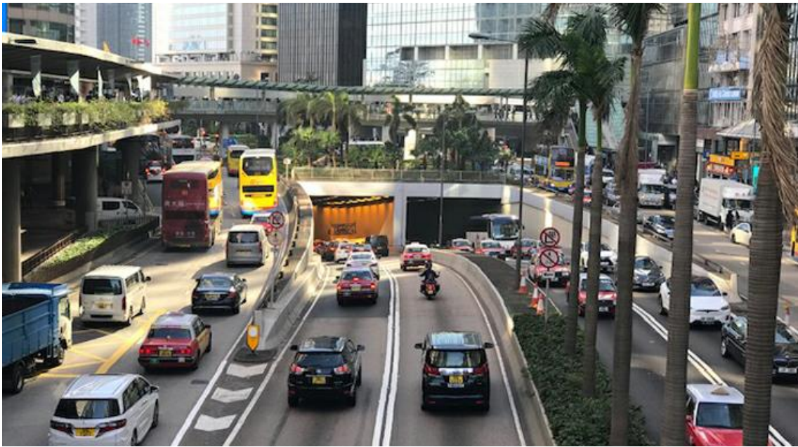
Figure 5.1(a): Connaught Road Central Underpass with AADT of 131,220
