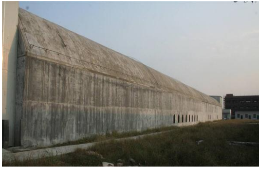
(a) External View of Test Tunnel
