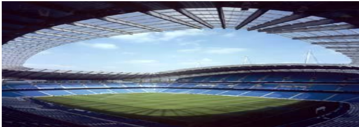
Figure 6.2 The City of Manchester Stadium interior (Photographer: Dennis Gilbert, architecture.com)
