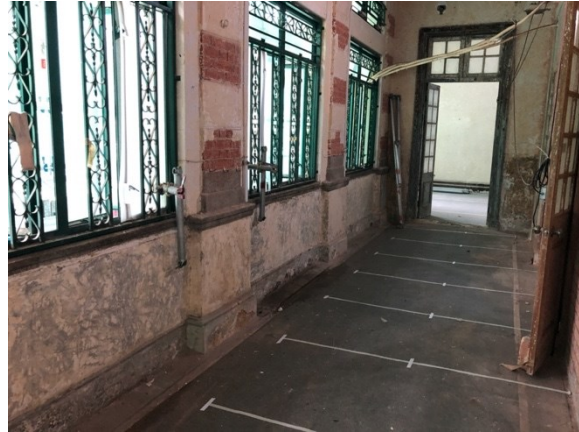
(b) Testbed 2 Corridor
