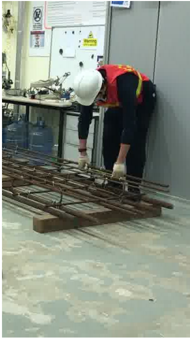
d. Measuring Rebar
