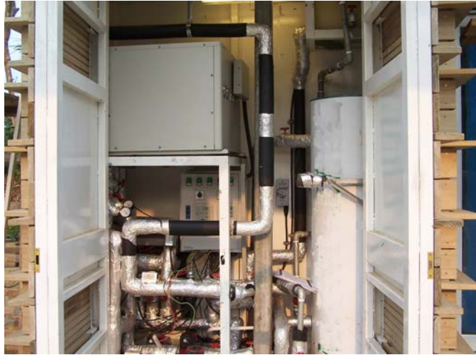
Figure 6.1 Photograph of the project
