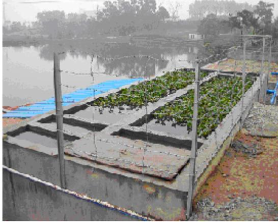
Fig. 3.2 Sedimentation tank
