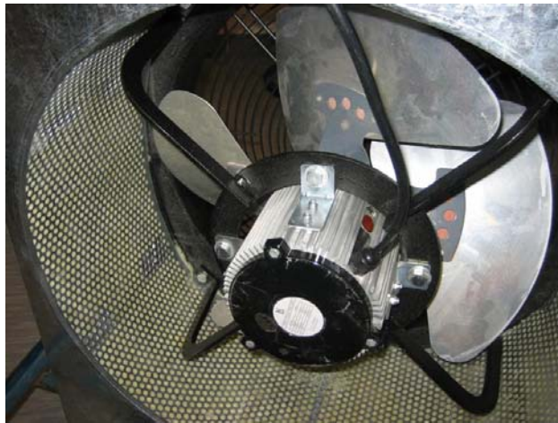
Figure 5.24: Propeller fan lining up with acoustic insulation
