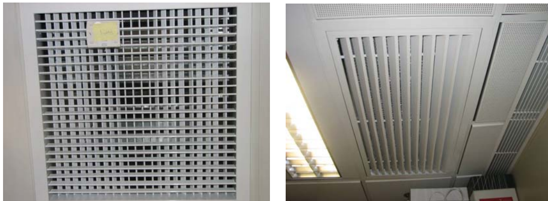
Figure 7.2: The geometry of the supply and return diffuser
