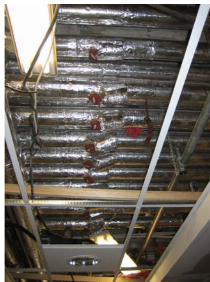
Figure 5.6: Chilled water pipe layout in the faculty office
