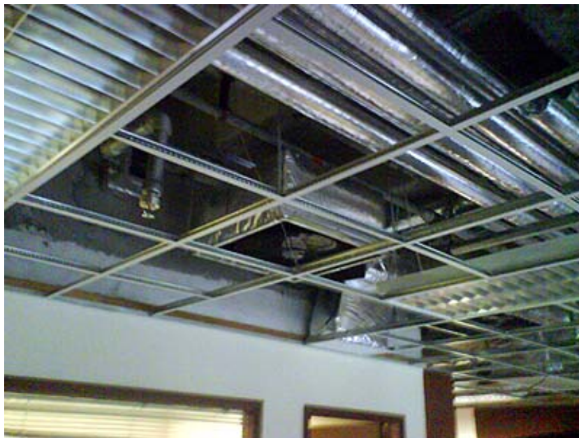
Figure 5.4: Internal wall up to the upper floor slab to reduce the latent load
