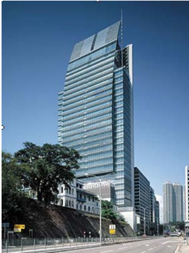
Figure 1.6 the PV facade of the building of One Peking
