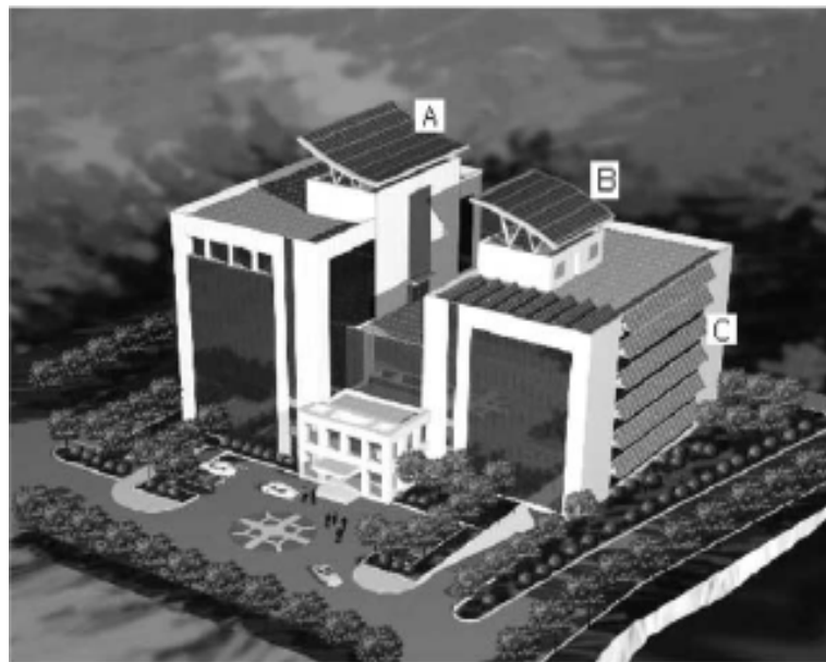
Figure 2.3 PV system of SIECT building
