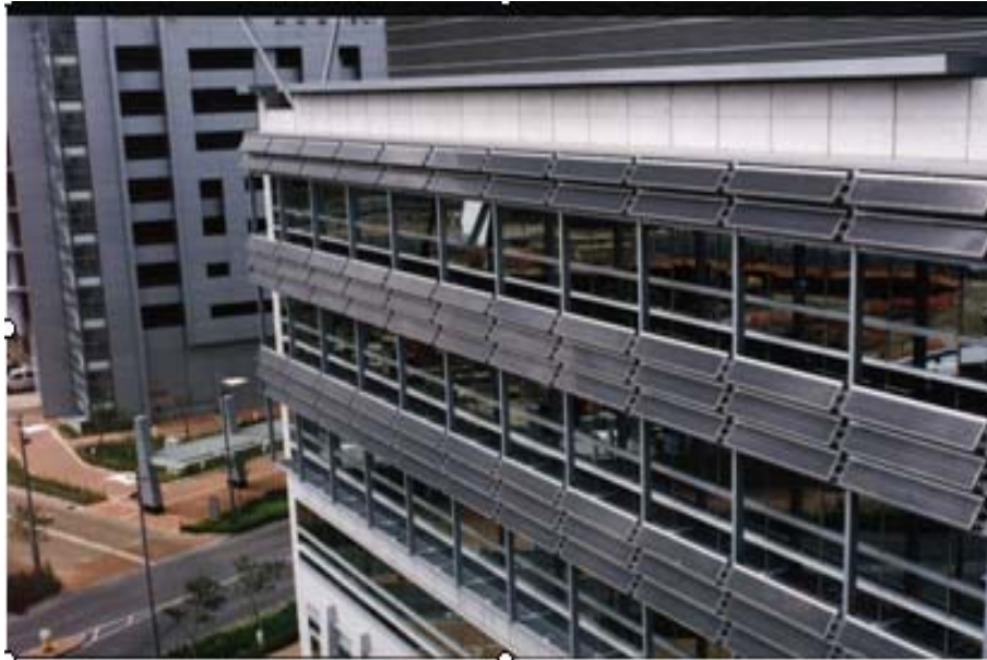
Figure 1.4 the Sun-shading system in the office building of Science Park
