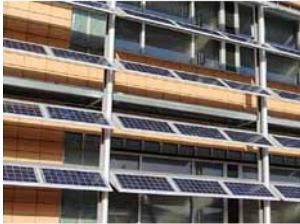
Figure 2.4 Sun-shading system of ECN building
