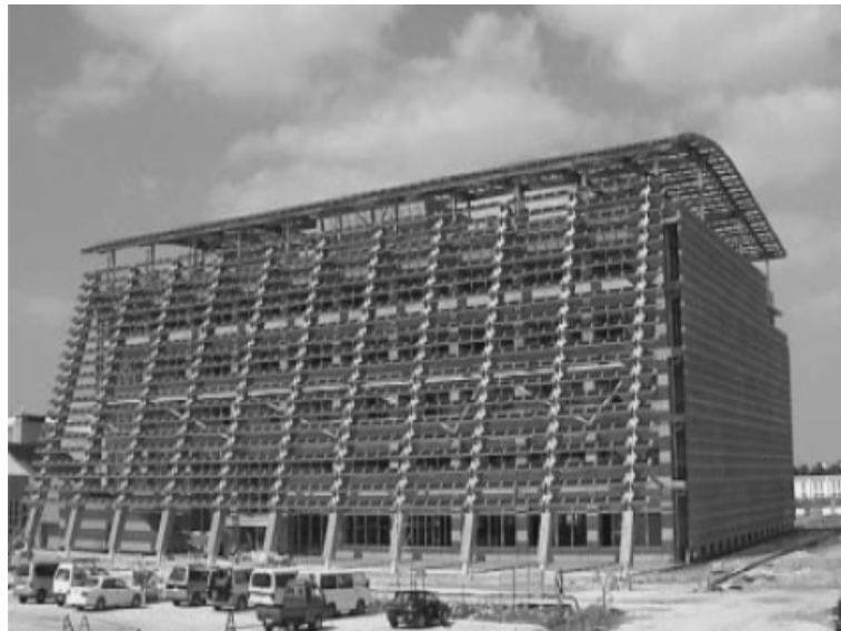
Figure 2.2 City Hall from the south
