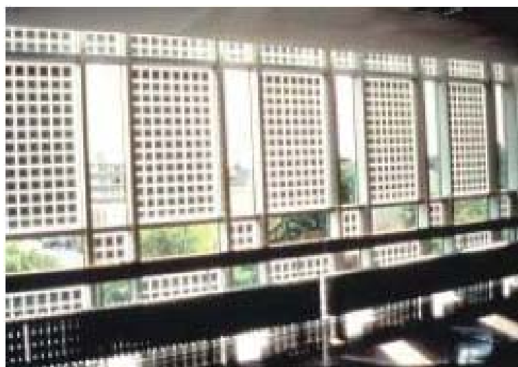
Figure 1.5 A semi-transparent BIPV facade
