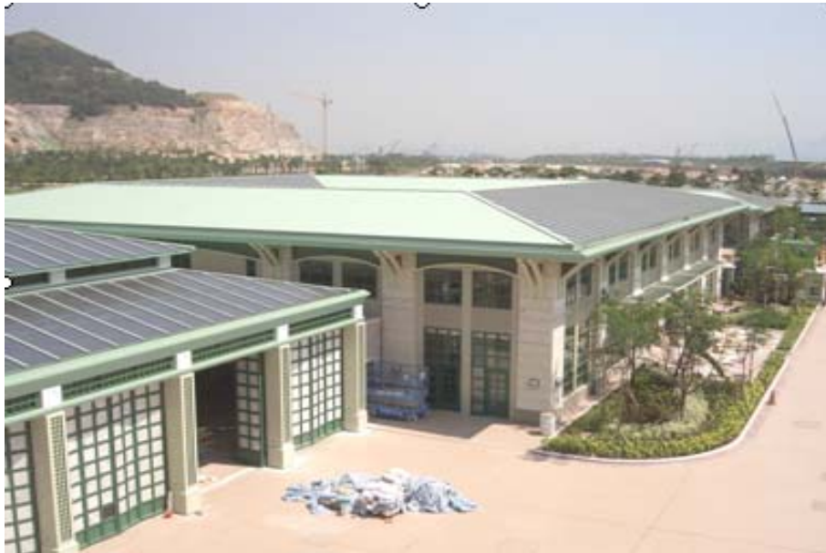
Figure 1.2 the PV roof in the office building of fire station in Penny Bay
