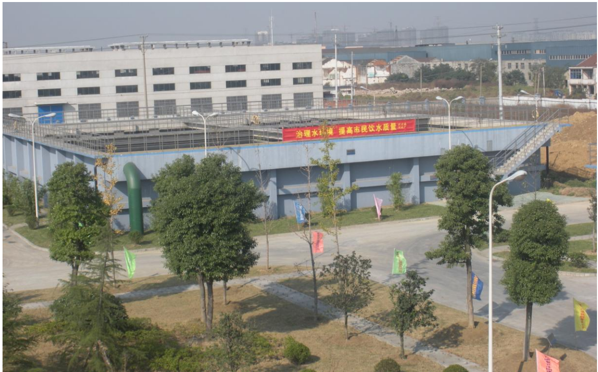
Figure 3.4 Anaerobic hydrolytic tank
