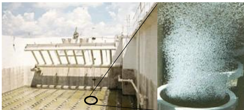
Figure 2.4 Batch tank with aerator and decanter devices
