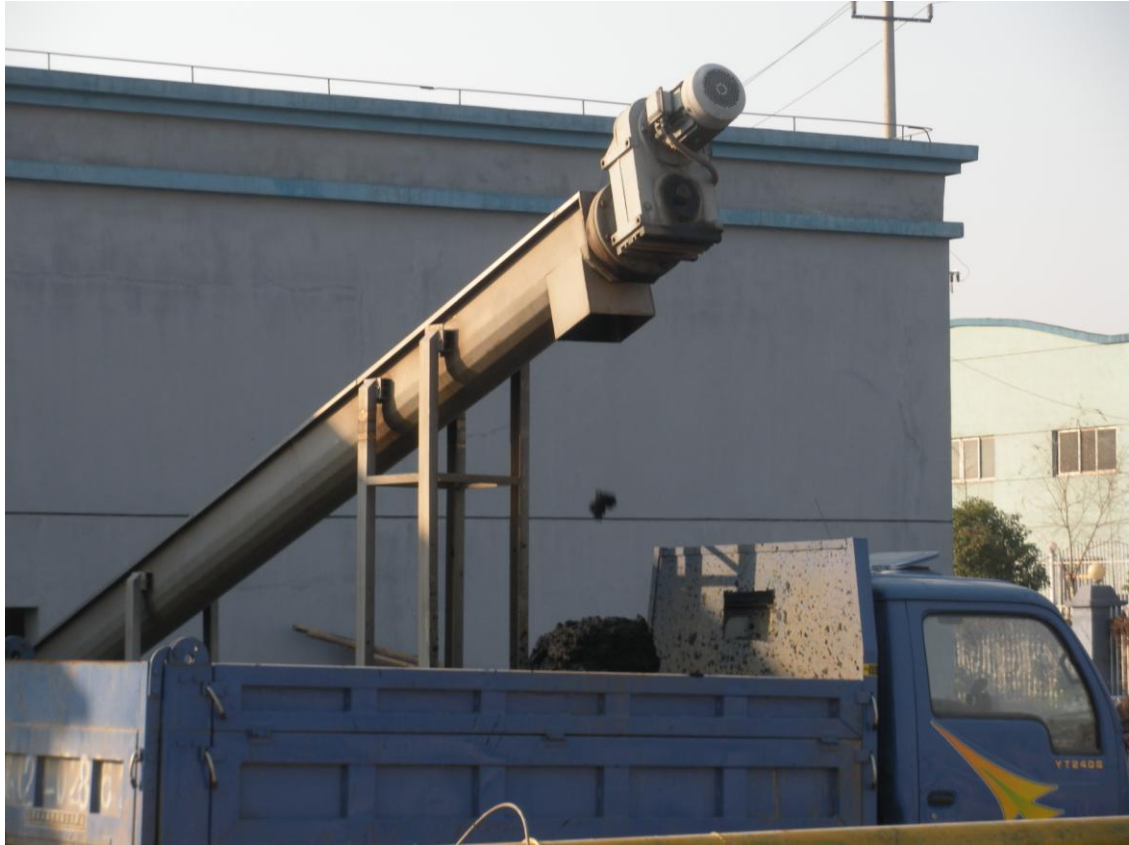
Figure 3.8 Sludge transporting after dewatering
