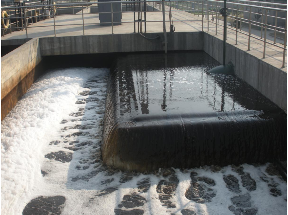
Figure 3.6 Biological selector in CAST sub-tank
