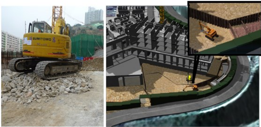
Figure 4.8 Visualized excavator operation versus the real excavation process
