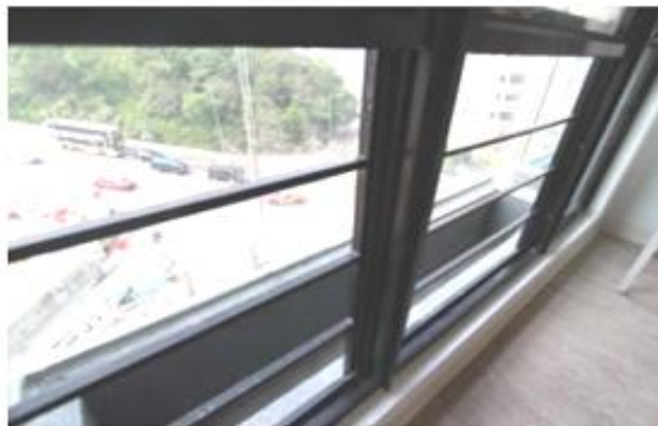
Figure 1: Photos of the new design single sided glazed ventilated window.
