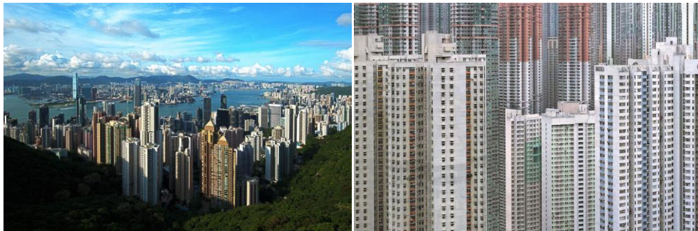
Figure 1- 1 High-rise buildings in Hong Kong.
