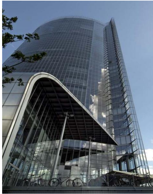
Figure 2- 20 Post Tower, Germany (King, 2012).
