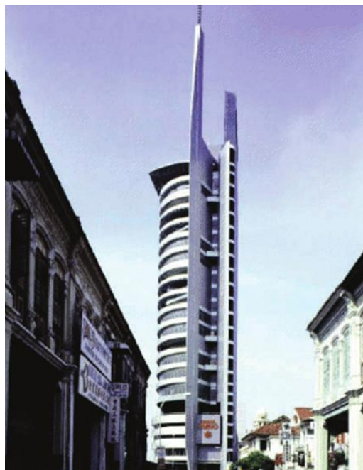
Figure 2- 15 Wing walls on the southeast of UMNO Tower.
