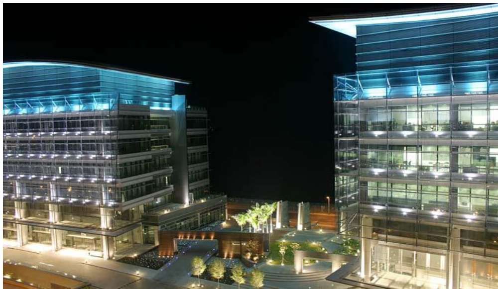
Figure 2- 9 Double-skin façade in Hong Kong Science Park.
