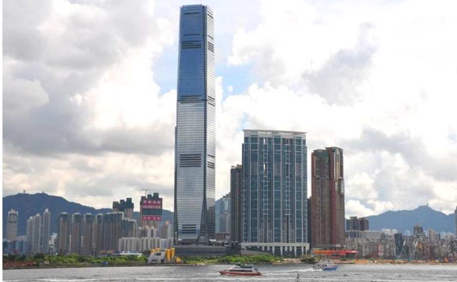
Figure 2- 5 Glass curtain walls of the International Commerce Centre (ICC) building.
