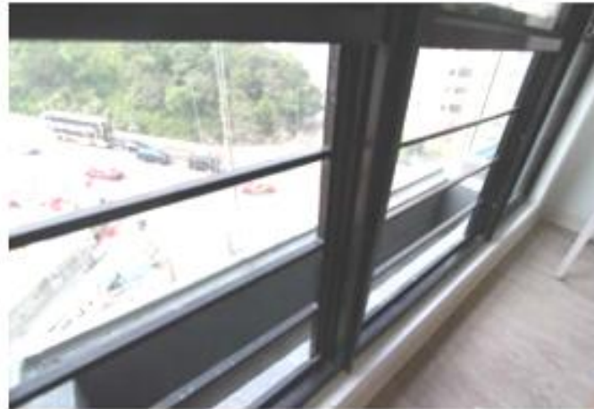
Figure 2- 10 Single-sided glazed ventilated window.
