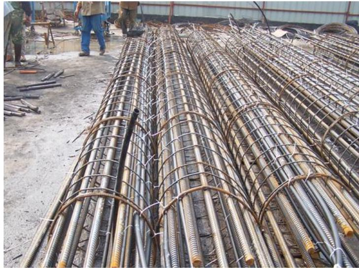
**Figure 2.1 The construction drawing of on-site pile foundation GHEs**
