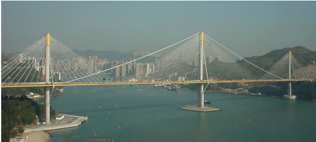
Figure 3.1 Ting Kau Bridge (TKB)
