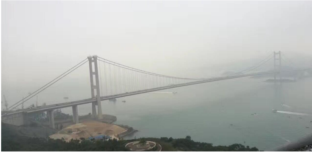
Figure 4.1 Tsing Ma Bridge (TMB)
