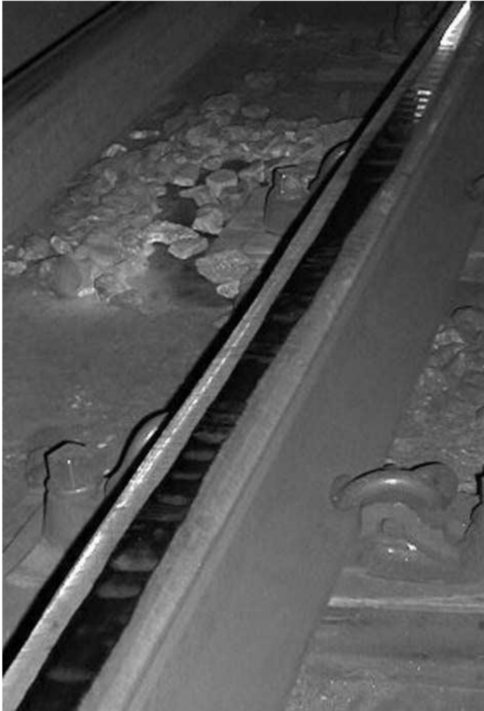
Figure 8. Pinned-pinned resonance corrugation on the rail[4]
