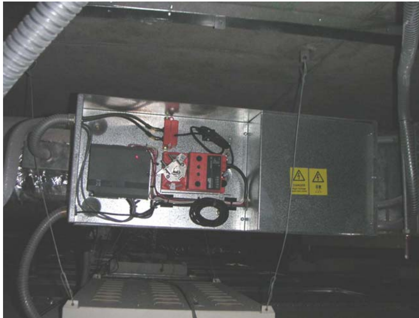
Figure 8.4 VAV terminal and its controller
