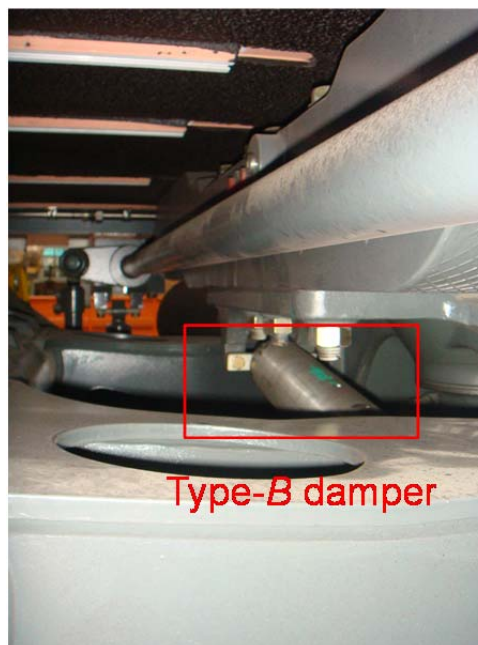
Figure 3.17 Laterally-deployed type-B MR damper in secondary suspension of tested EMU train vehicle
