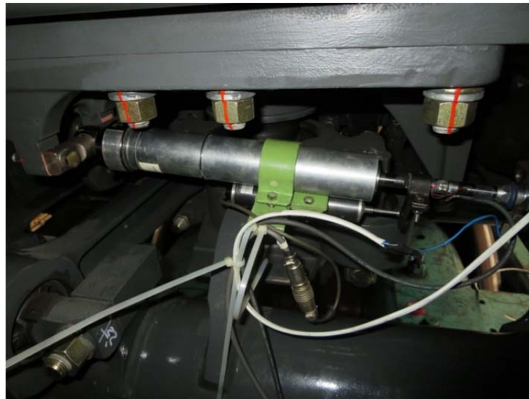
Figure 4.3 Installation of MR damper
