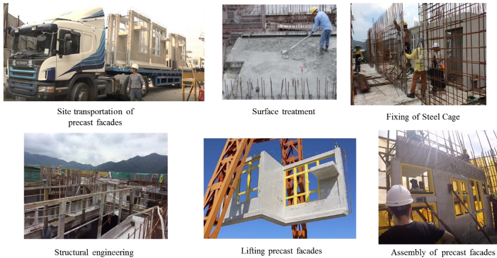
Figure 4.15 On-site construction process
