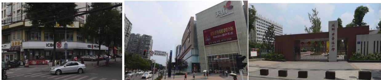
Figure 4. 10 Photos of Jinyang neighbourhood infrastructure
