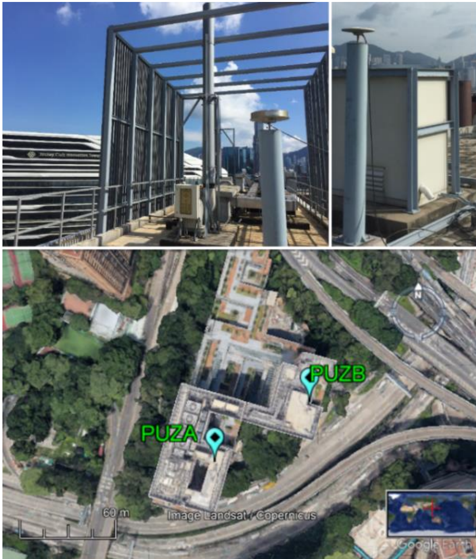
Figure 5-3 Multi-GNSS sites PUZA (up left) and PUZB (up right) with a distance of approximately 50 m
