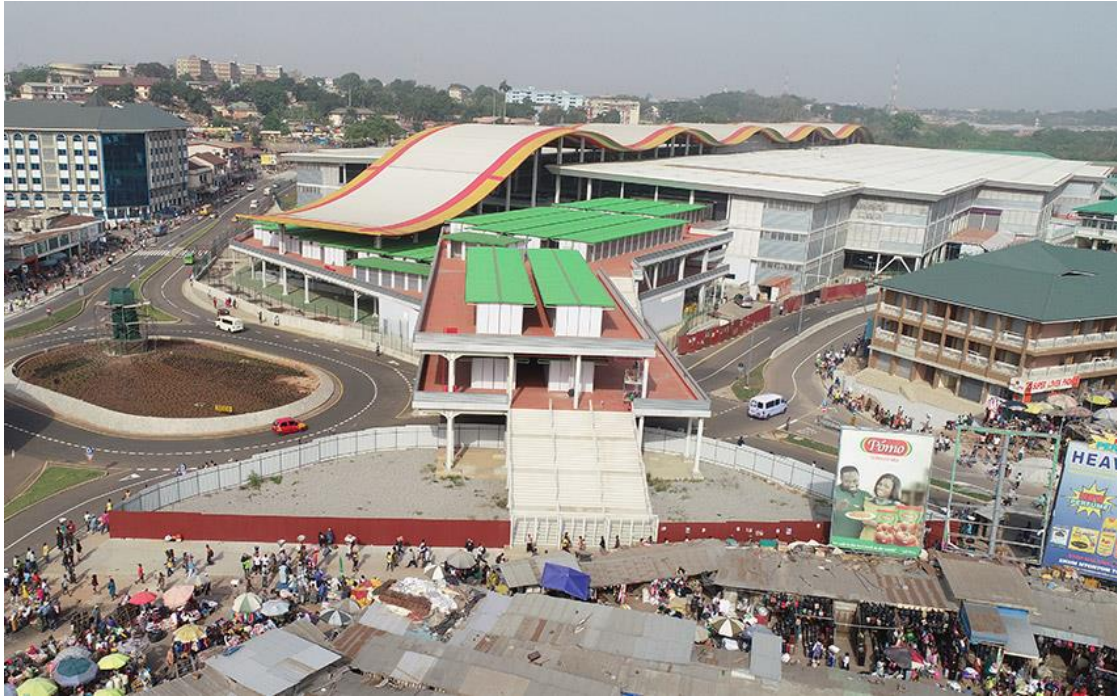
Figure 8.10 First phase of redevelopment project completed
