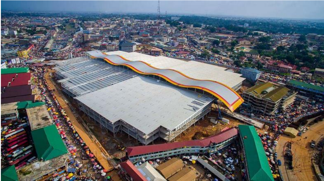
Figure 8.9 First phase of redevelopment project in execution
