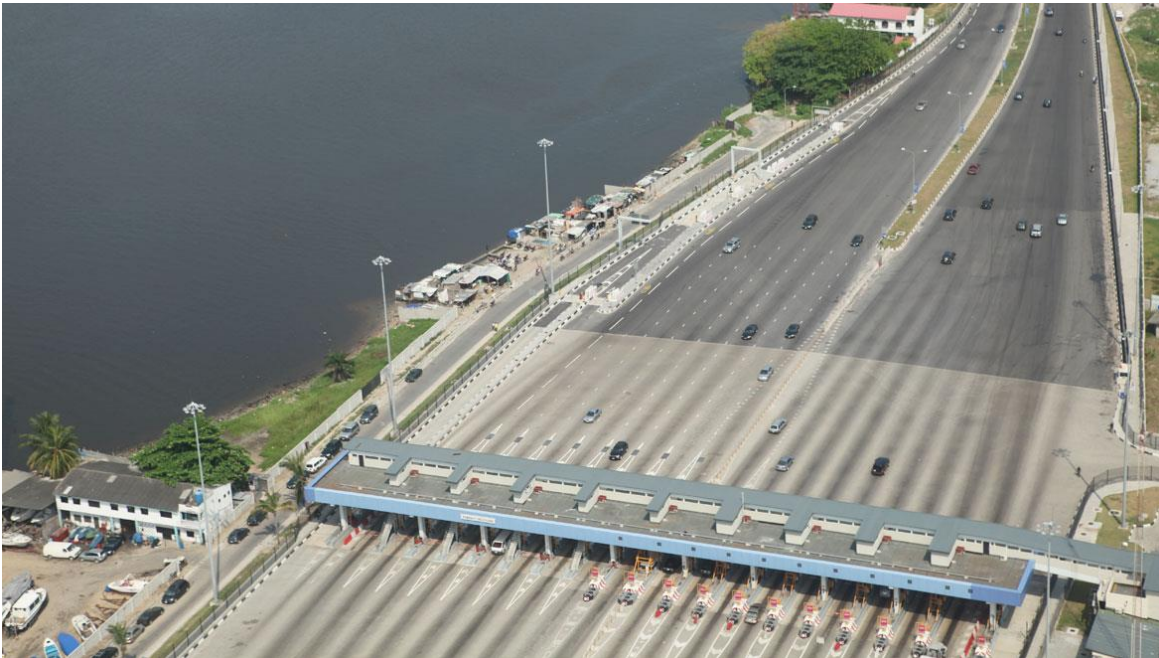
Figure 4.1 Nigeria Lekki toll road concession project
