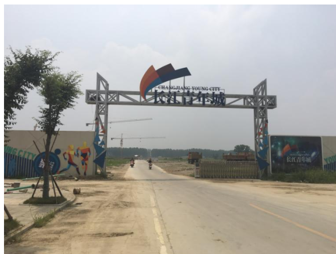
Picture 5.7 Construction Site of Affordable Housing Project
