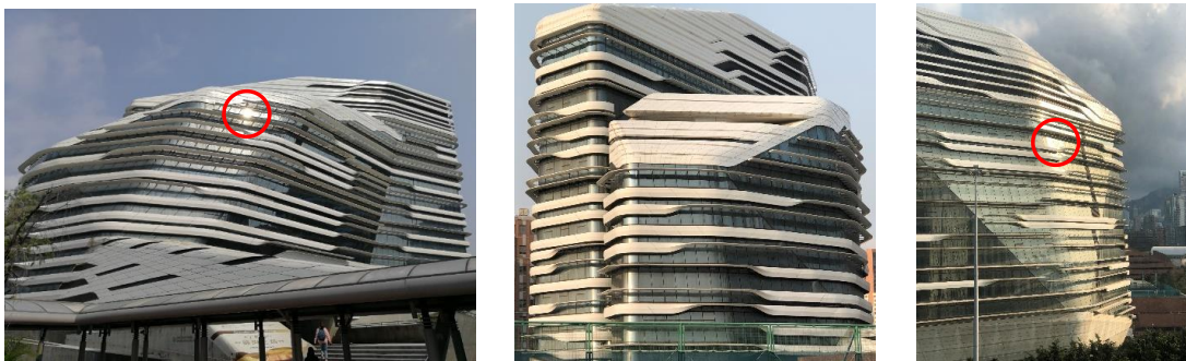
Figure 7.1 Photograph of the Jockey Club Innovation Tower in The Hong Kong Polytechnic University, with the red circles highlighting the reflected sunlight from the curtain wall.
