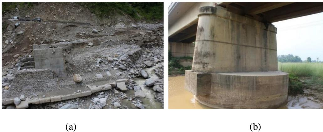
**Figure 2-2** (a) Collapsed and washed away bridge due to 2017 flood in Nepal and (b) scouring observed in a bridge in Nepal after the 2017 central Nepal flash flood (photos adapted from (Li *et al.* 2020a)).
