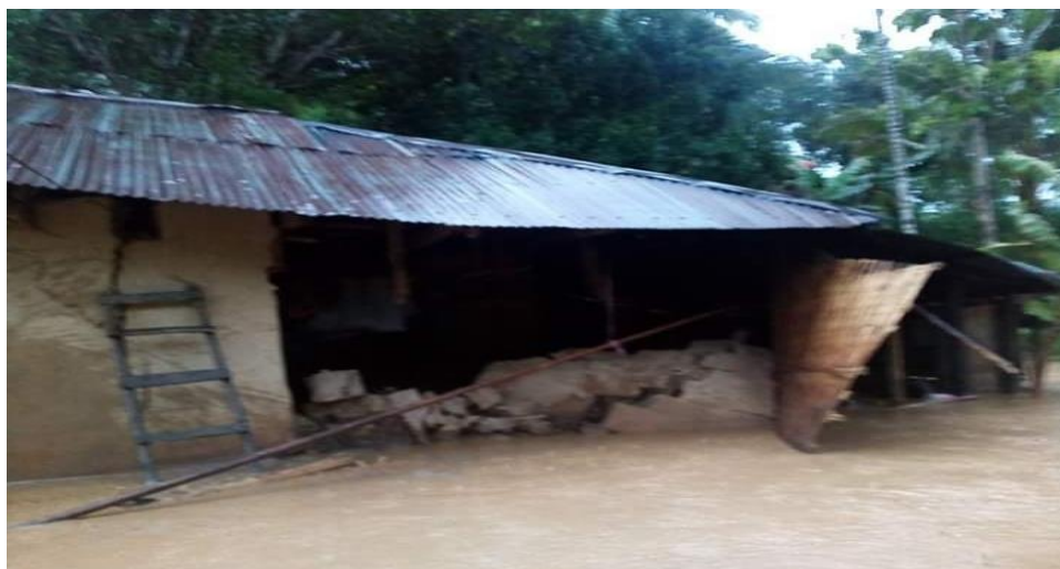
Picture 4.3: Flood water damages houses
