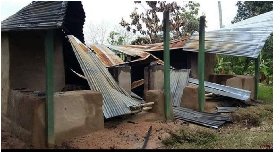
Picture 4.4: Cyclone damages houses in CHT
