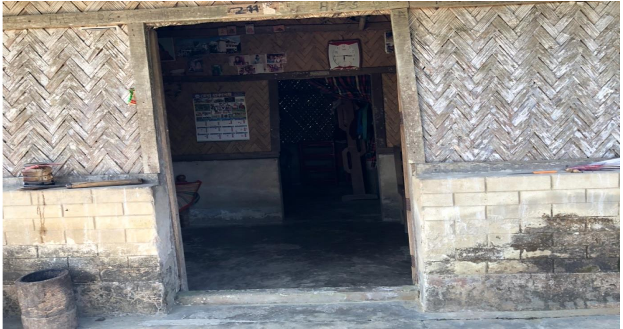
Picture 5.1: Make temporary wall with this door to prevent flood water to enter room during flood
