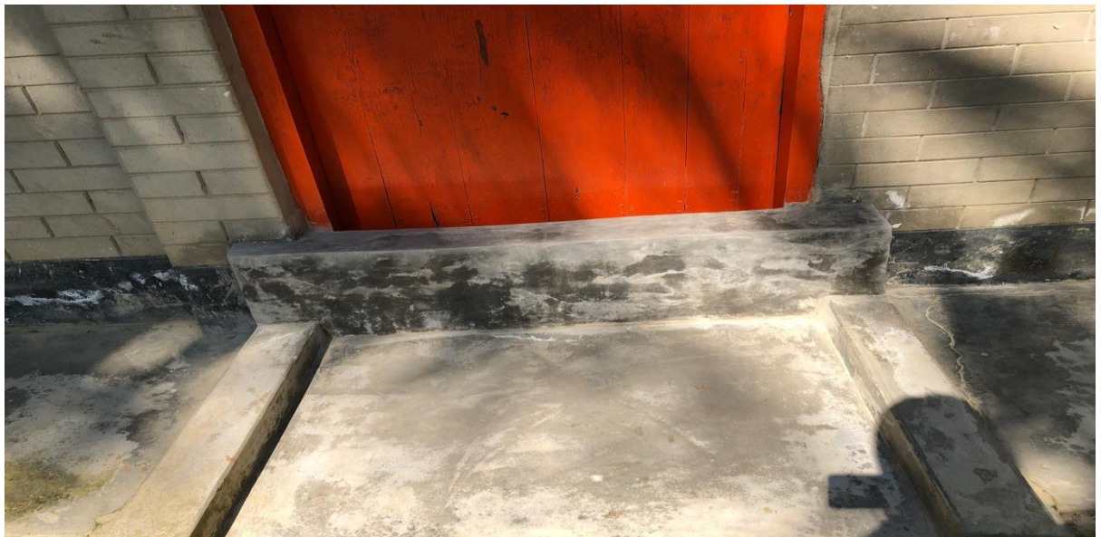
Picture 5.2: Make small wall to this door to protect flood water to enter room during flood
