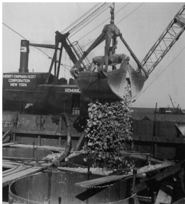
Figure 2.2 Construction of Mackinac Bridge (ACI 304.1)
