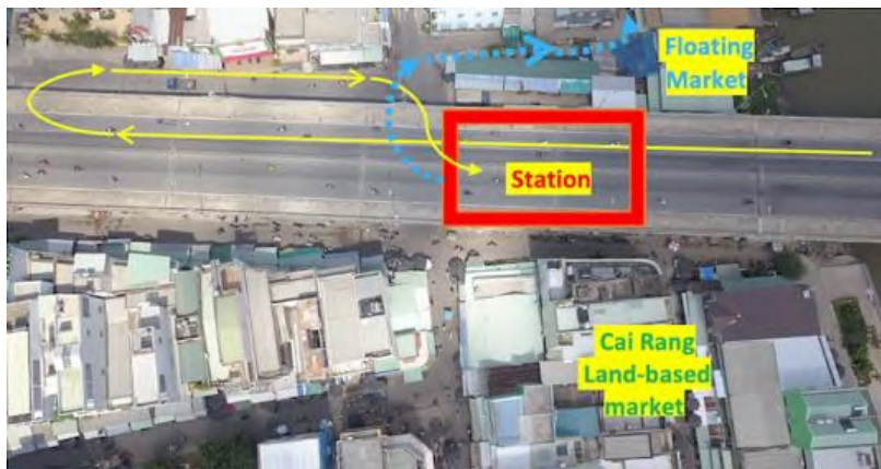
Fig. 5 & 5a: Aerial view of the Cai Rang bridge and boat drivers' station
