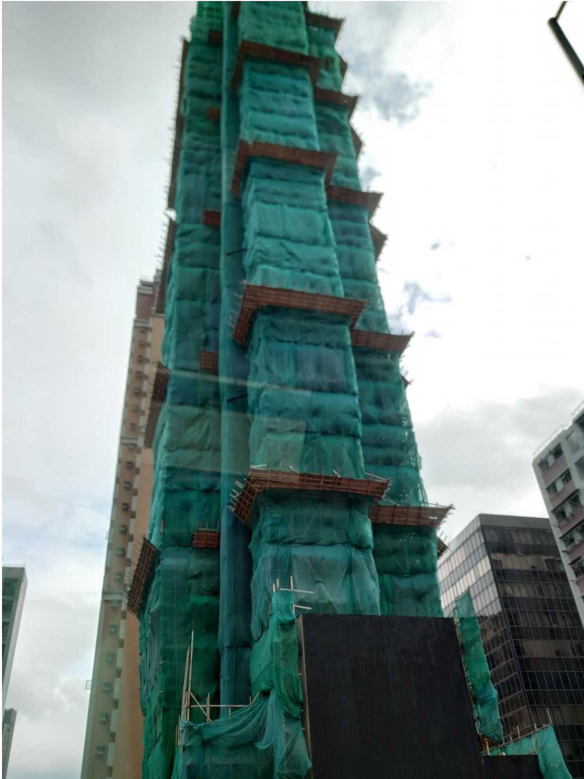
Figure 4-46 Bamboo scaffolding around buildings for construction purposes (photo by Anthony)
