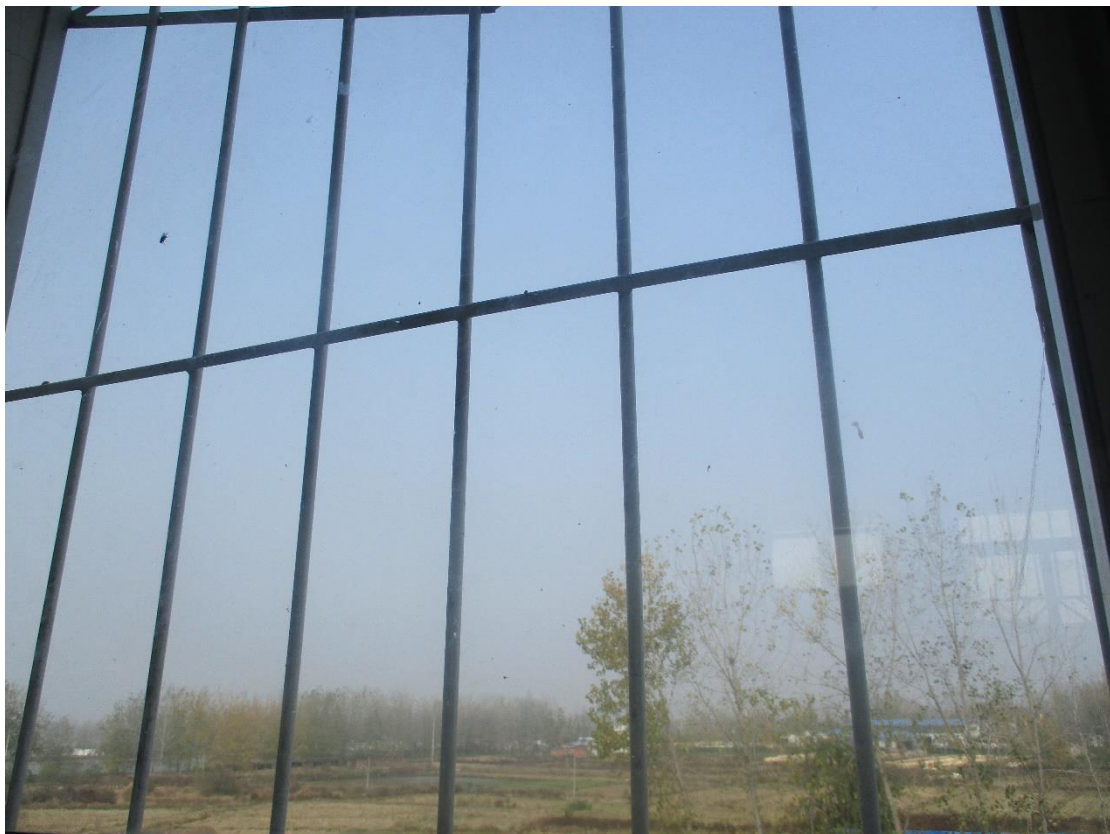
Picture 8. The window bars (taken by Bei Bei)
