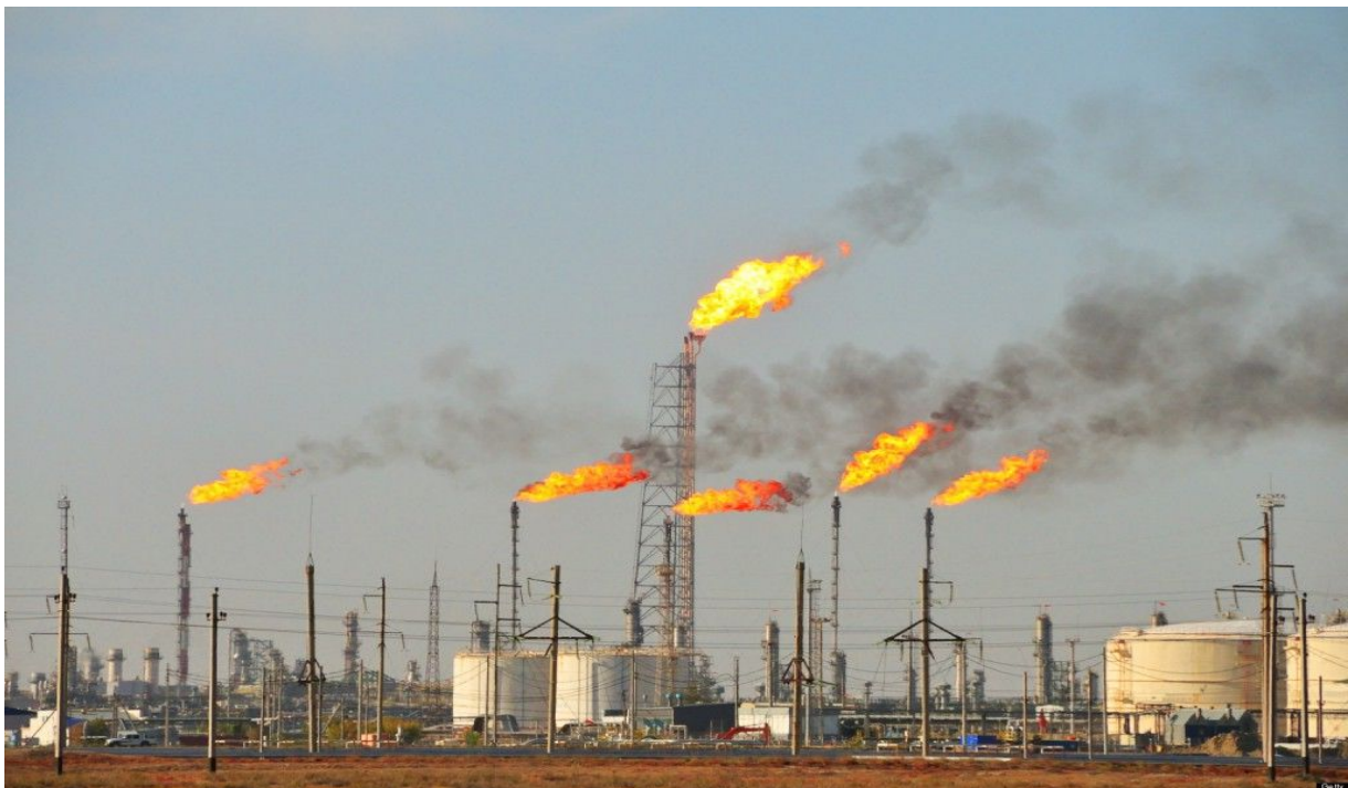
Figure 1.2: A typical gas flaring site in Southern Nigeria (Source: Aggreko)
