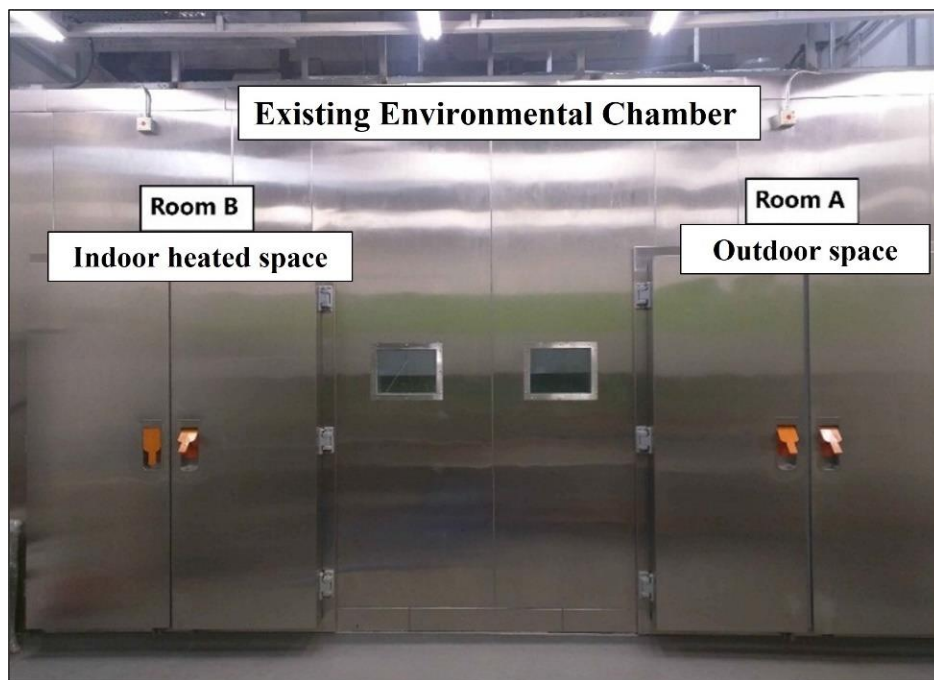
Photo 4 The existing environmental chamber
