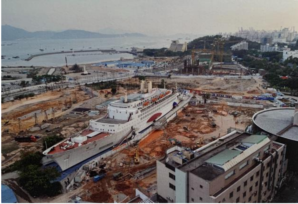
Figure 29. The Mingwah liner and the Sea World area under construction in 2012.
