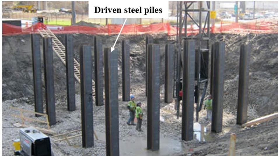
Figure 2.3 Driven steel piles in the ground at site ([shortspansteelbridges.org](http://shortspansteelbridges.org))
