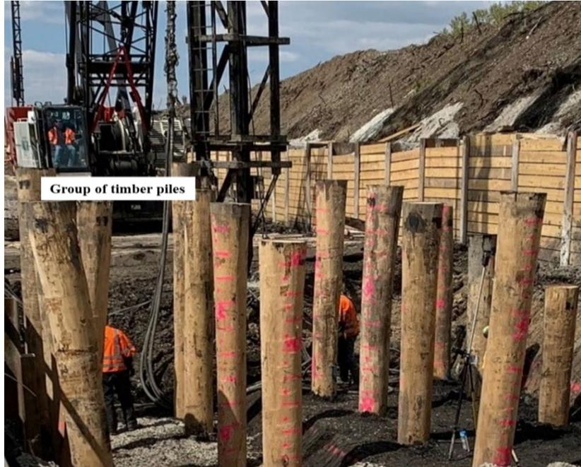
Figure 2.7 Group of driven timber piles in ground (weekesforest.com)
