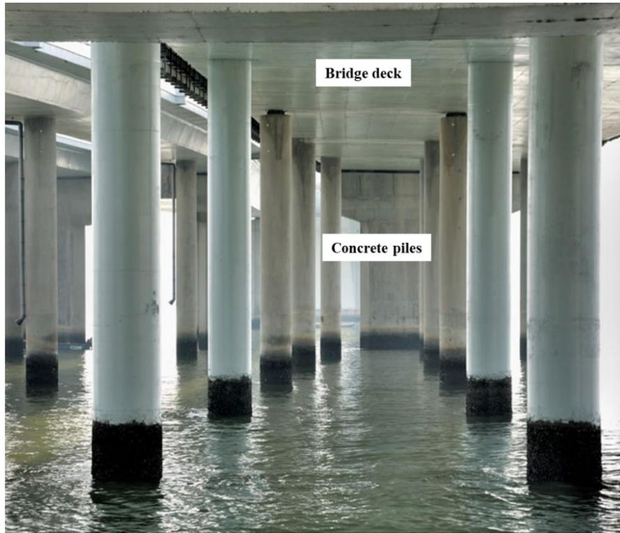
Figure 2.5 Offshore concrete piles (pilebuck.com)
