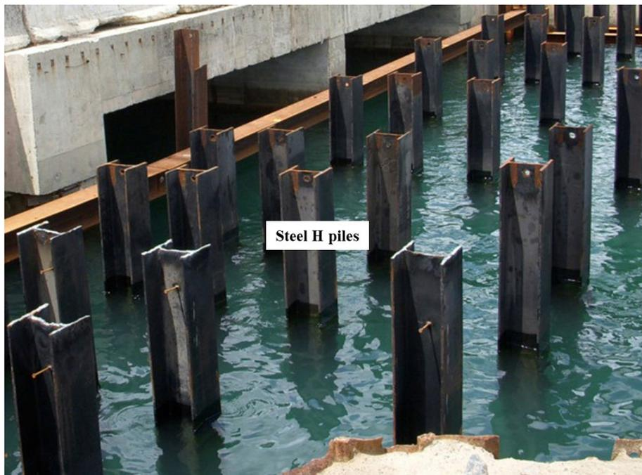
Figure 2.6 Group of offshore H shaped steel piles (morrisshea.com)
