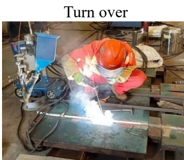
d) Manual welding for the 1 st pass
