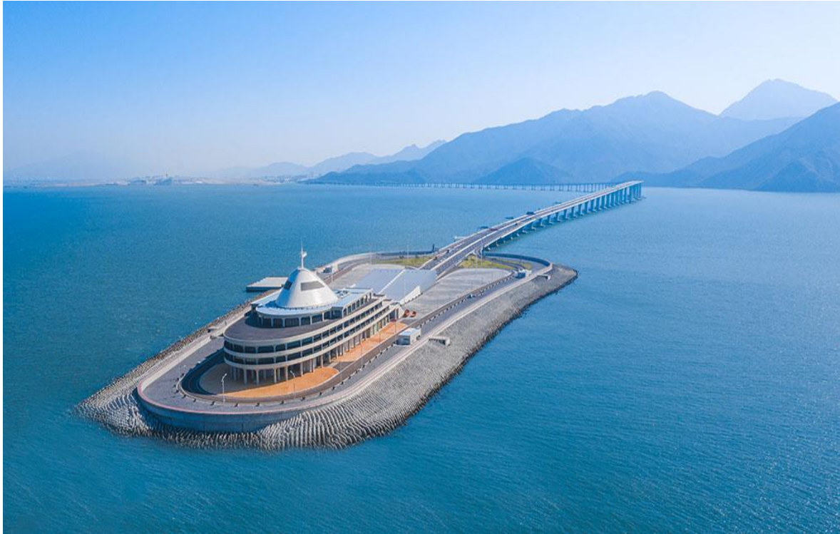
(b) Artificial island of the Hong Kong-Zhuhai-Macao Bridge
