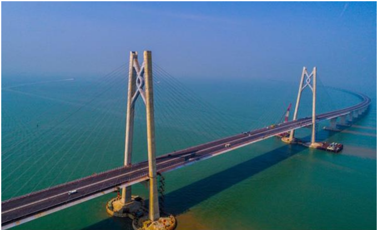
(a) The Hong Kong-Zhuhai-Macao Bridge under construction in April, 2017
