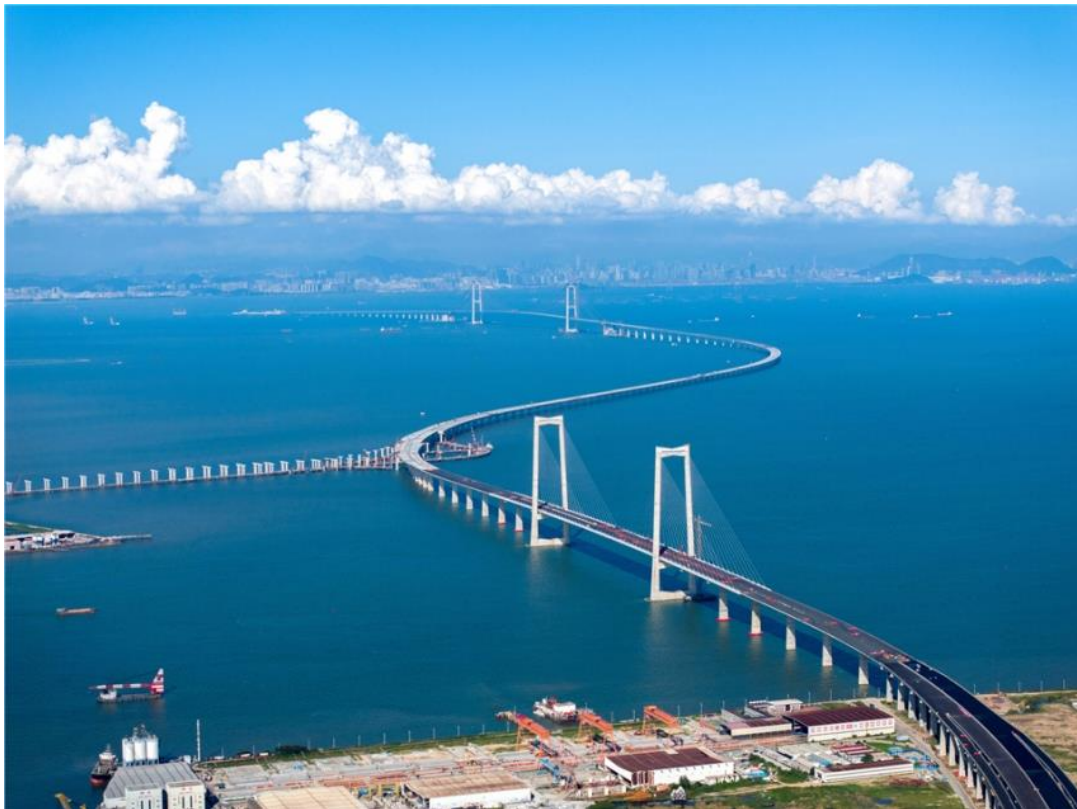
(b) Real scene picture of Shenzhen-Zhongshan Bridge Tunnel Link
