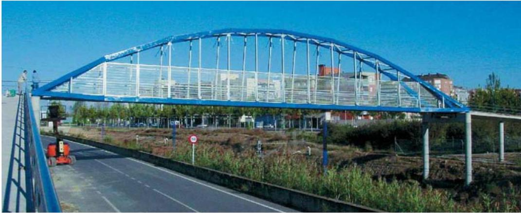
Figure 2.5 Footbridge made of GFRP pultruded profiles in Lleida, Spain (Hollaway, 2013)
