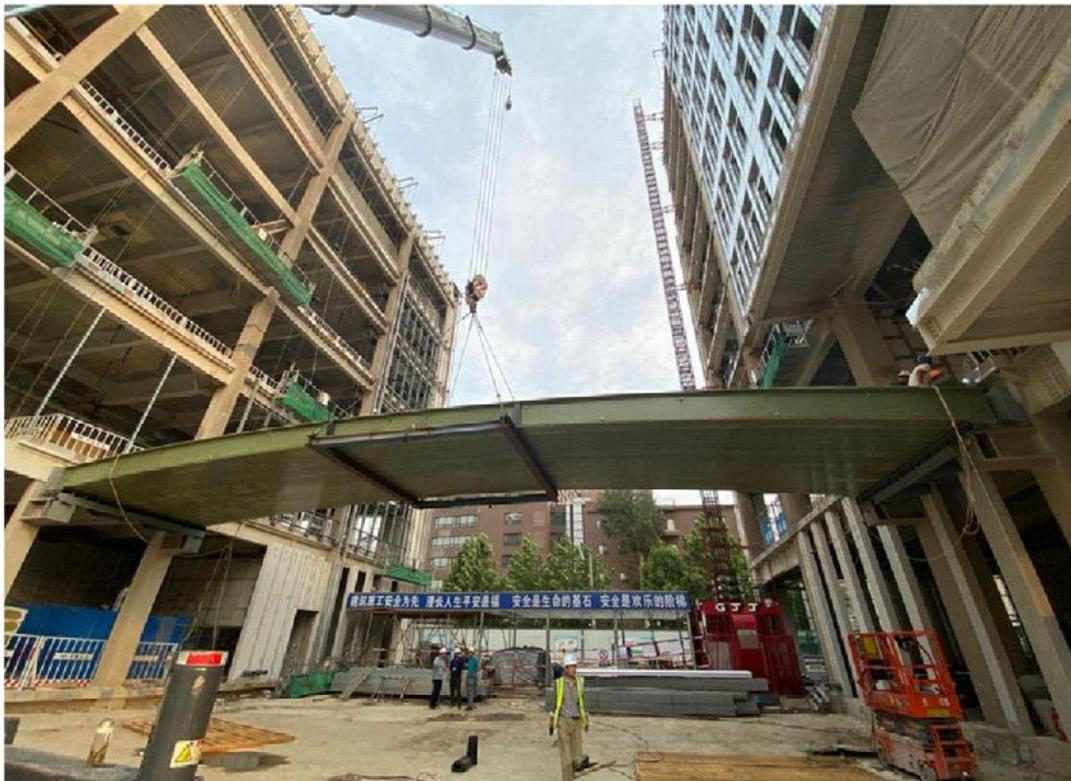
Figure 2.6 Curved-pultruded GFRP footbridge in Beijing, China (Liu et al., 2021)
