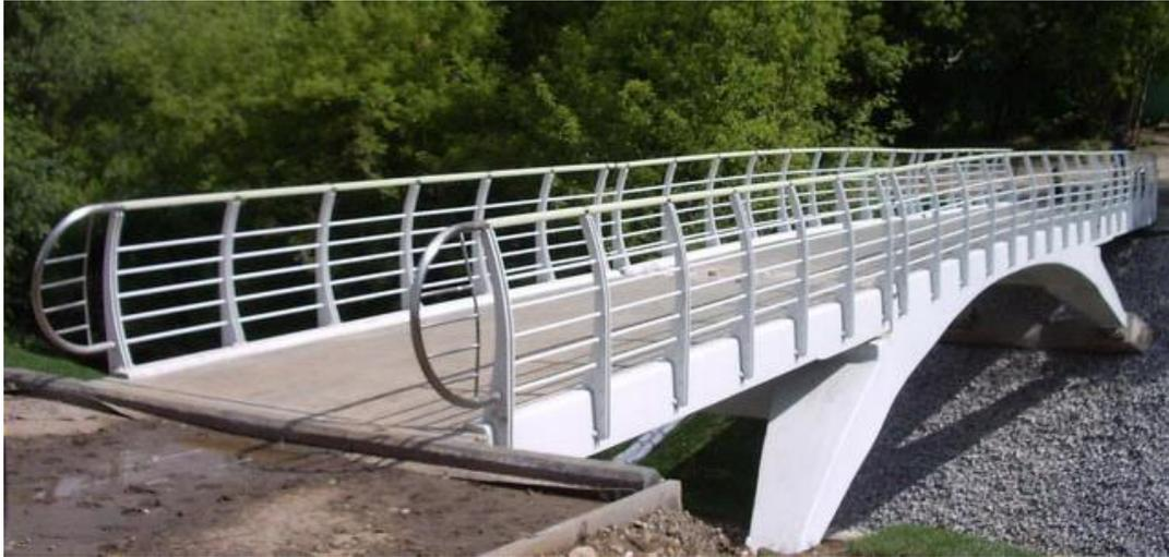
Figure 2.7 Footbridge manufactured by vacuum infusion in Moscow, Russia (Hollaway, 2013)
