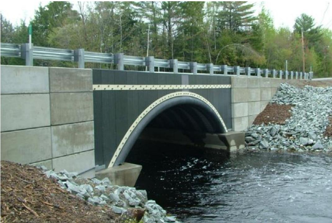
Figure 2.13 Buried CFFT arch bridge in Maine, USA (Dagher et al., 2012)
