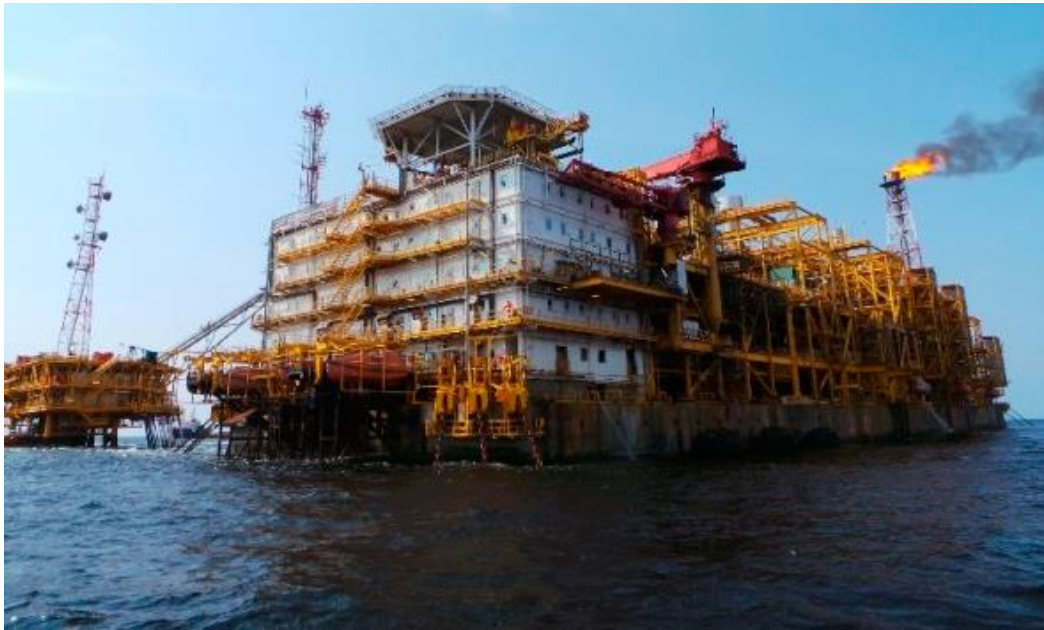
Fig. 2.5. N’Kossa floating prestressed concrete barge (Source: Oil&Gas Journal 2019)
