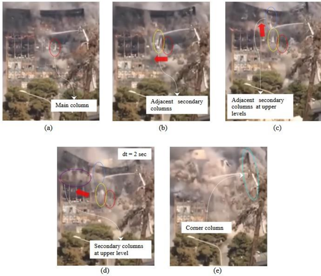
Figure 7.37 Collapse sequence observed in video evidence 3
