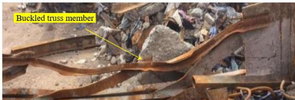
Figure 7.18 Buckled truss beam found in debris
