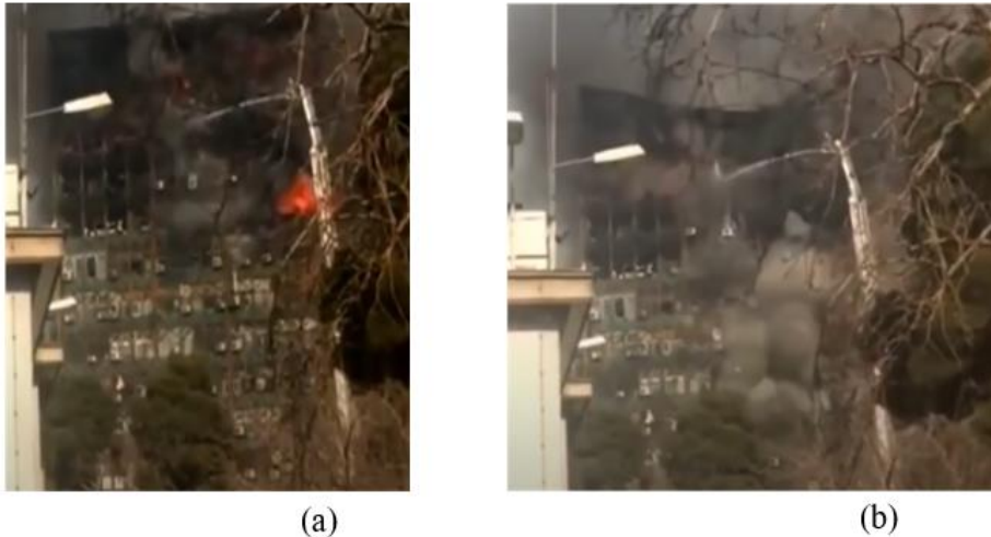
Figure 5.35 Screenshots (a) and (b) from video evidence show the South side peripheral column being pulled inwards seconds before the tower collapses.
