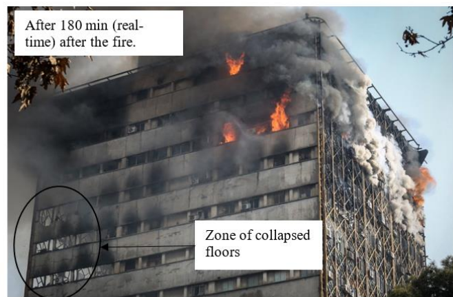
Figure 6.16 The photo shows the loss of fire-affected corner floors while the tower still stood.
