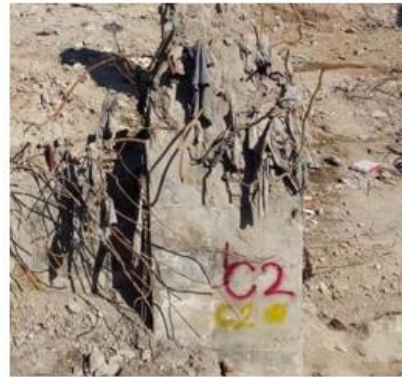
(b) A marked location for extracting concrete sample
