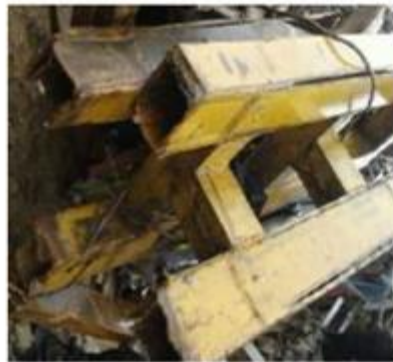
(c) Photo of collapsed corner column
