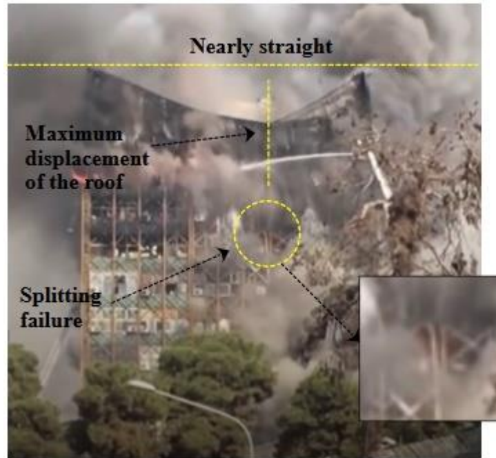
Figure 7.32 A significant moment during the global collapse
