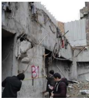
(a) Survey of the location and dimensions of surrounding walls.
