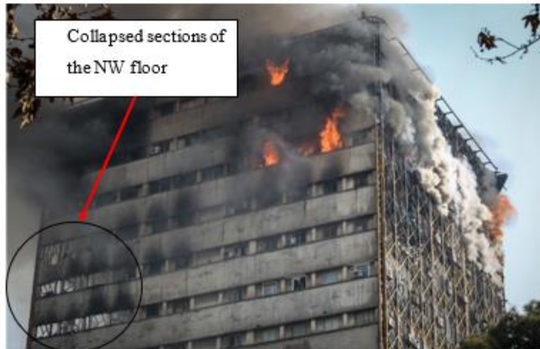
Figure 3.1 Photo showing the partially collapsed floors in the NW corner of the tower (West elevation)
