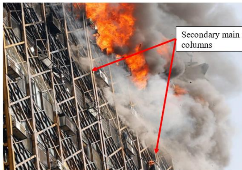
Figure 3.14 Photo of the tower showing fire possibly heating two primary beams simultaneously.
