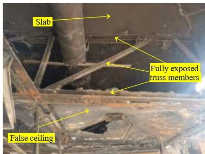
Figure 7.9 Photo showing the fully exposed steel members (Shakib et al. (2020))
