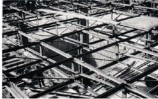
(a) Photo of the floor truss system taken during the construction stage.
