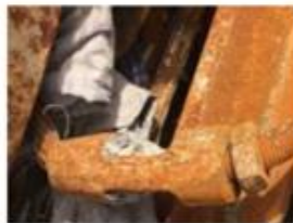
(c) Bolted connection in the debris
