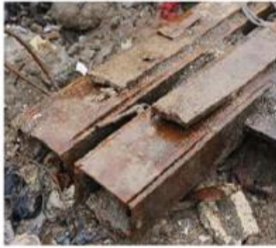
(a) Photo of collapsed main secondary column
