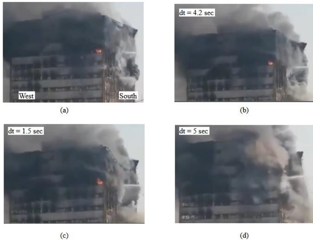
Figure 7.35 Collapse sequence observed in video evidence 1
