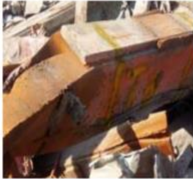
(c) Photo of collapsed minor secondary column
