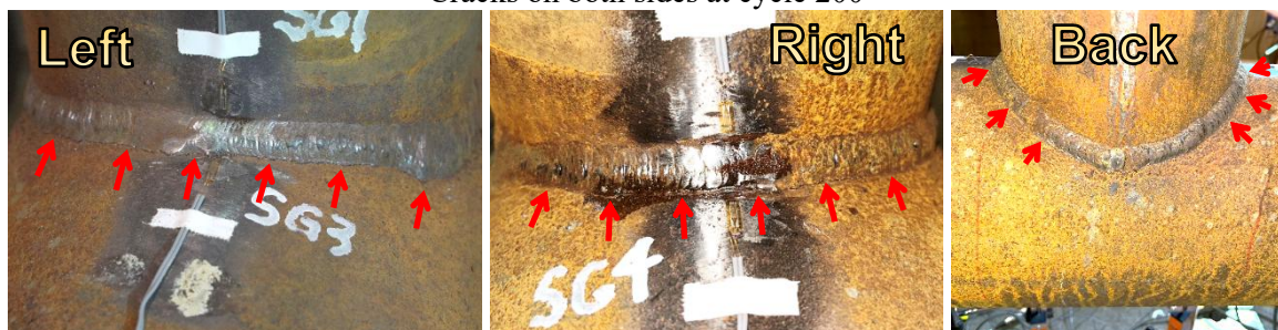
Obvious cracks on both sides at cycle 259
