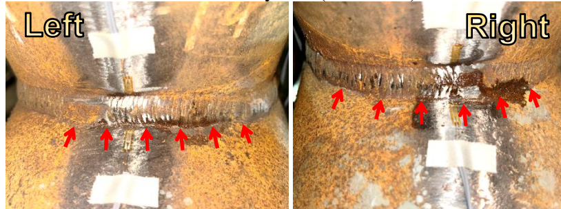
Crack initiation on both sides at cycle 5
