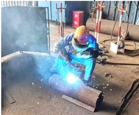
c) Welding of steel tubes
