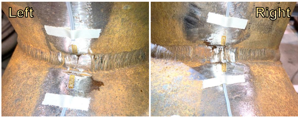
No crack on both sides at cycle 0 (before test)
