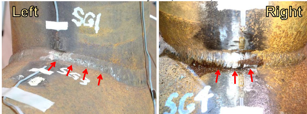
Crack initiation on both sides at cycle 9
