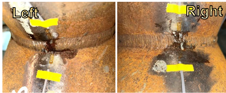
No crack on both sides at cycle 0 (before test)
