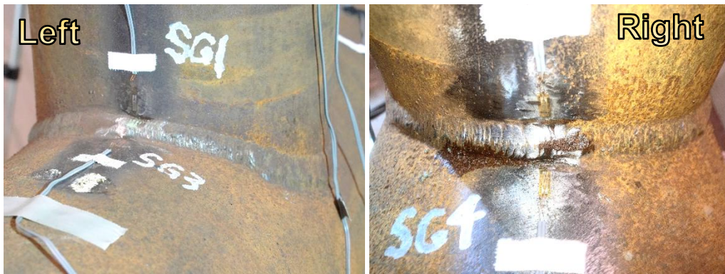
No crack at cycle 0 (before test)
