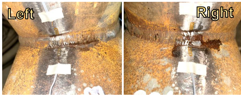
No crack at cycle 0 (before test)
