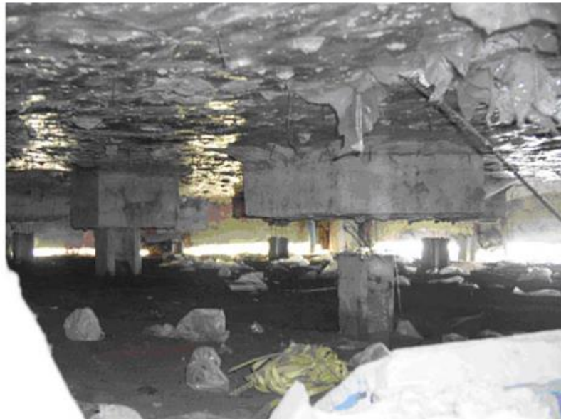
Figure 2-9 Field case of piles dragged down from the pile cap due to negative skin friction (after Su et al. 2020)
