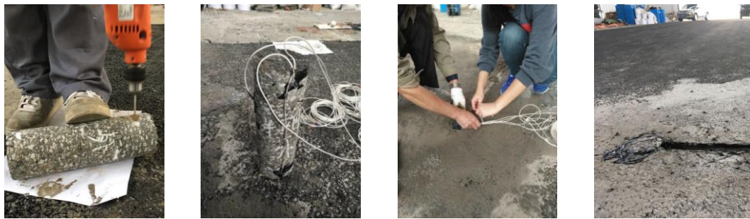
(a) Coring and drilling
