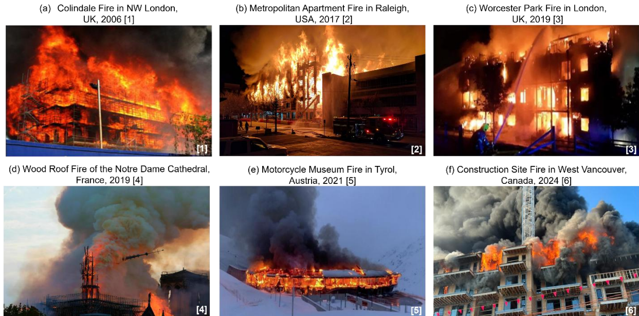
Fig. 1.1. Fire accidents in timber buildings: (a) Colindale Fire in NW London, UK, 2006 [1]; (b) Metropolitan Apartment Fire in Raleigh, USA, 2017 [2]; (c) Worcester Park Fire in London, UK, 2019 [3]; (d) Wood Roof Fire of the Notre Dame Cathedral, France, 2019 [4]; (e) Motorcycle Museum Fire in Tyrol, Austria, 2021 [5]; (f) Construction Site Fire in West Vancouver, Canada, 2024 [6].
