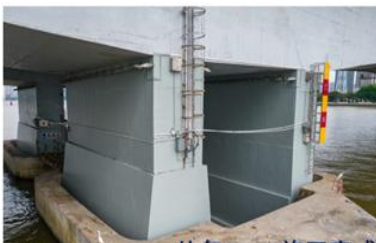
(c) Bridge pier reinforcement.
