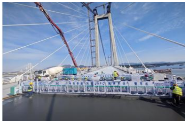
(a) Bridge deck pavement.
