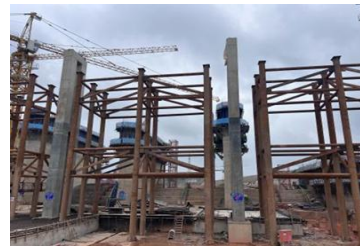
(b) Bridge pier components.
