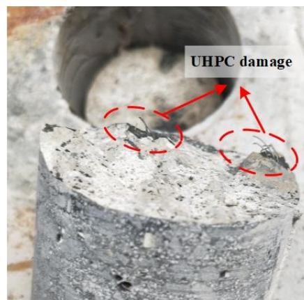
Figure 7.13. NC-UHPC tensile failure surface.
