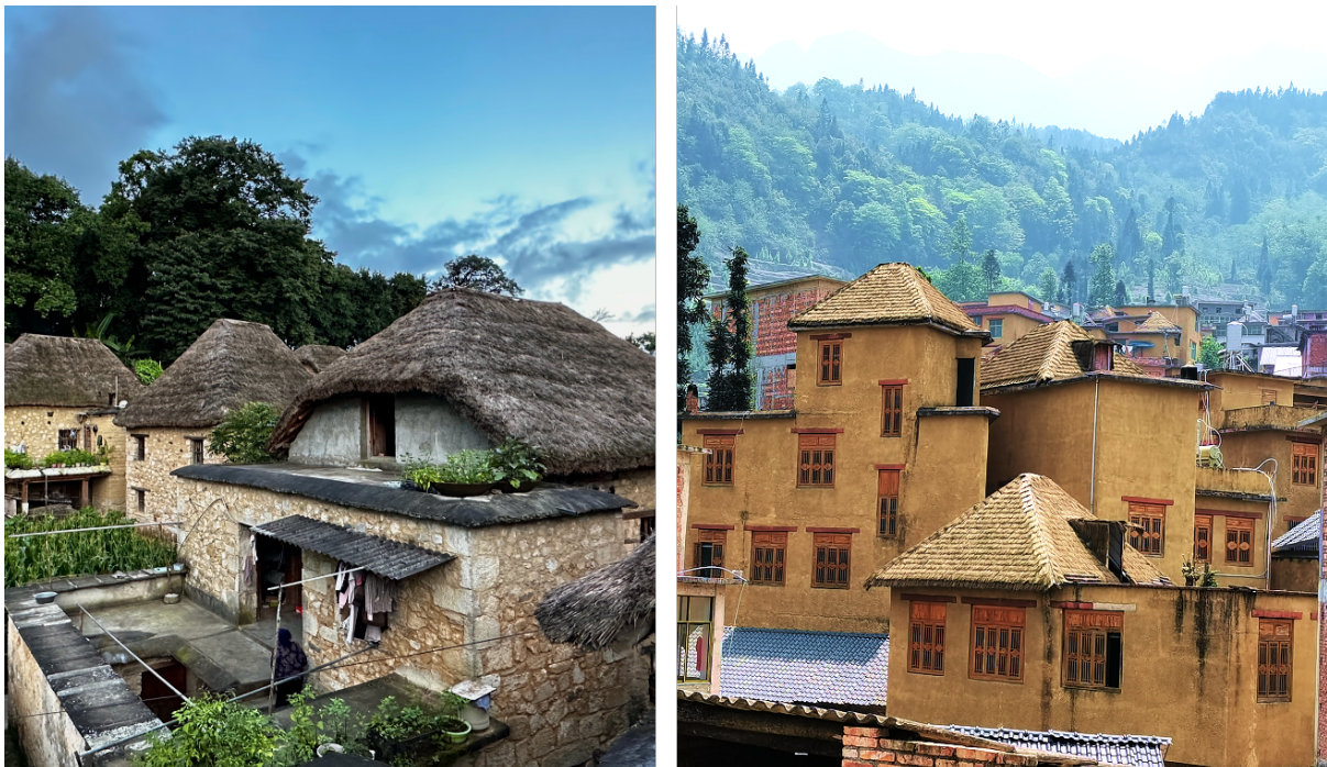
Figure 16. Demolition and reconstruction in Azheke (left) and Duoyishu (right) villages
