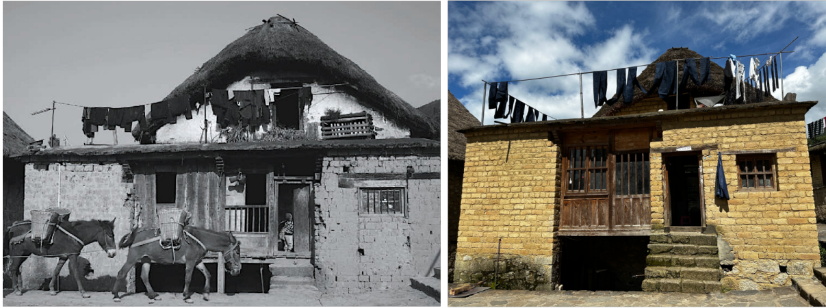
Figure 15. Demolition and reconstruction in traditional style in Azheke village
