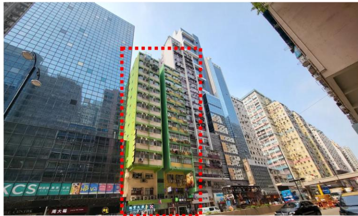
Actual location of the case study building
