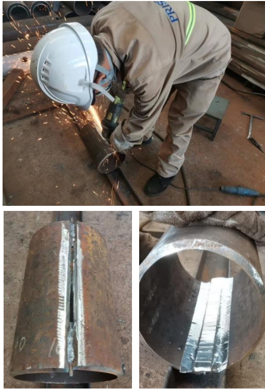
a) Preparation works
