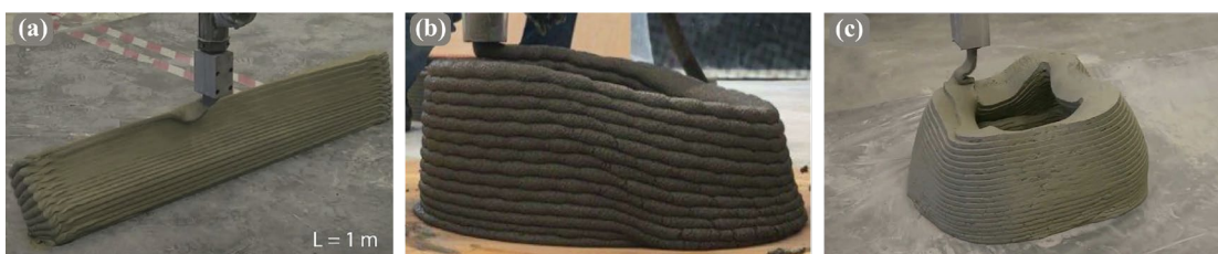
Figure 1.3 Failure of 3D-printed structures during construction: (a) A free-standing wall [extracted from Wolfs et al. (2019)]; (b) A cylindrical wall [extracted from Jayathilakage et al. (2020)]; (c) A rectangular wall [extracted from Suiker et al. (2020)].
