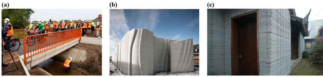
Figure 1.1 Examples of construction projects utilising the extrusion-based 3D concrete printing technology: (a) 3D-printed bicycle bridge at the Eindhoven University of Technology [extracted from Salet et al. (2018)]; (b) 3D-printed IT server hotel by COBOD [extracted from Symonenko (2024)]; (c) 3D-printed Chinese courtyard by WinSun Limited [extracted from WinSun (2015)].
