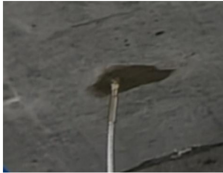
Figure 6-13 Sensor probe fixed with quick hardening cement
