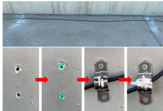
Figure 3-6 Armored fiber cables fixed on the ground
