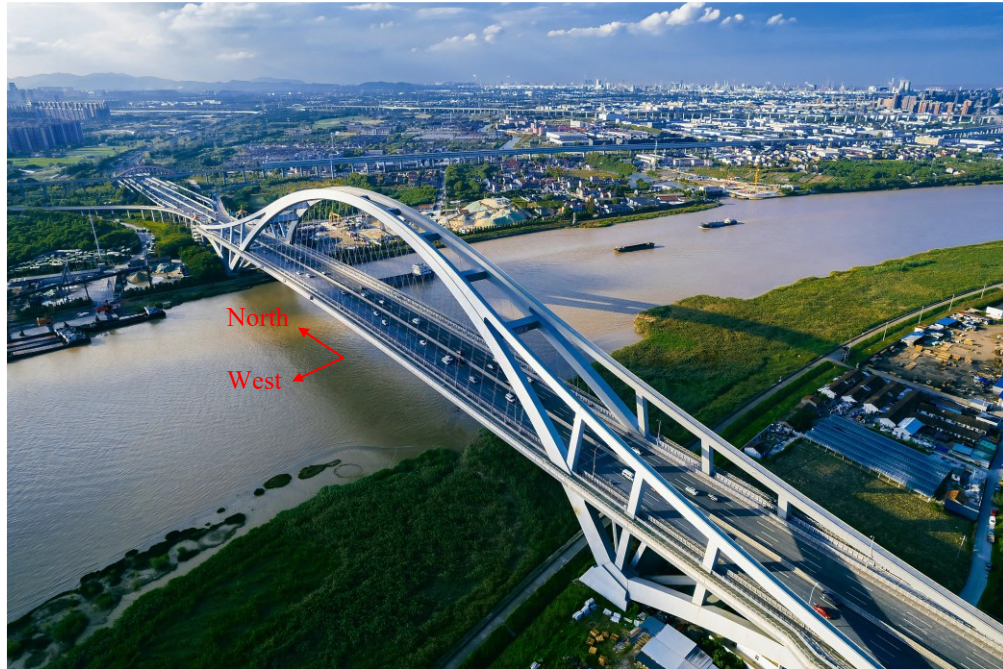
Figure 5.2 Southwest view of the Mingzhou Bridge
