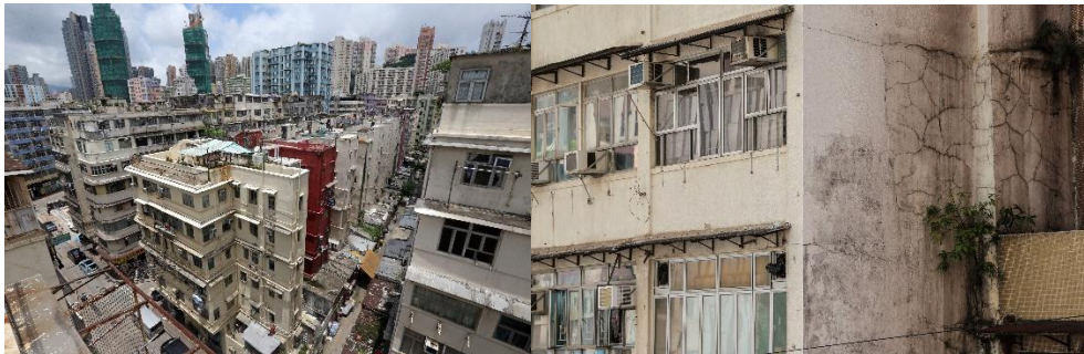
Fig. 1.1 Examples of aging buildings in Hong Kong.
