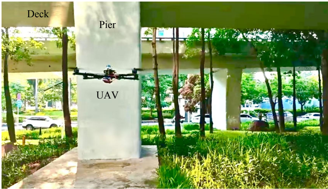
Figure 5.9: The UAV is flying around the bridge piers and deck for coverage inspection task.
